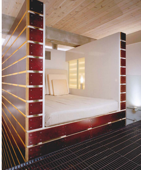
Square-head screws, all turned in the same direction, fasten the barn boards to the MDF panels. Painting the panels white allowed the specialty lighting within the router-cut ½-inch grooves to reflect off the panels, enhancing hallway light and providing reading light.
